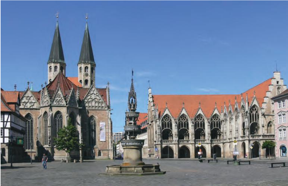
Fig. 3 The old market place of Braunschweig. From left: the clothiers' Guild Hall, the Martini Church and the Old Town Hall. All these medieval buildings are made of red rogenstein from the Nussberg.
